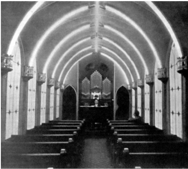
In 1898 Daniel McFarlan Moore created a model of a stone church he named the Moore Vacuum Tube Chapel and inside held a wedding, dramatically lit by vaulting arcs of white Moore tubing.
