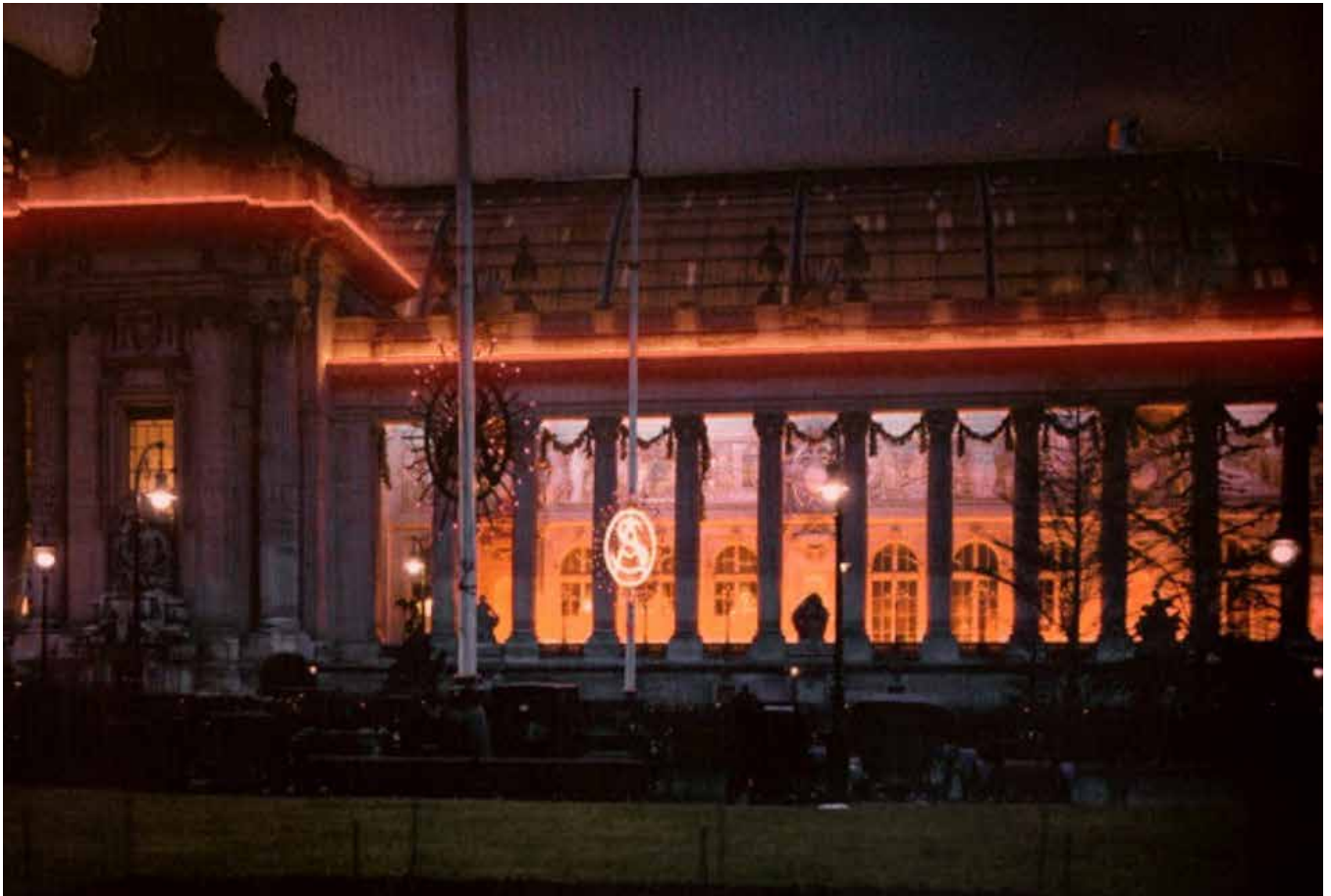
In 1910 Georges Claude used Moore tubing filled with neon to light the exterior of the Grand Palais des Champs-Élysées for the Paris Salon de l'Automobile.
