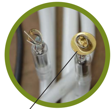
Use brass electrode buttons to increase connectivity.
