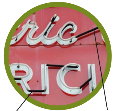
Block-out paint should be applied to define letter forms and tube ends. Eventually this paint will peel off and should be reapplied.
