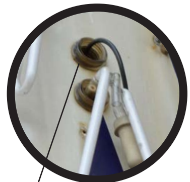
Never run wire from the exposed electrode into a hole/glass housing.
