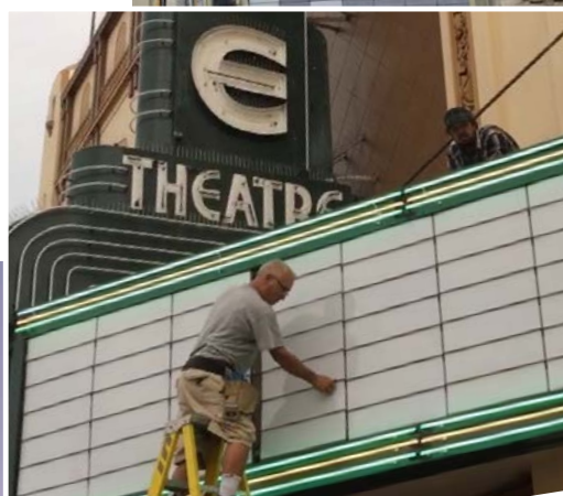
Photo: Randall Ann Homan 2017, Avenue Theater, San Francisco, CA L-R, Jim Rizzo and Nate Macie putting the final touches on the marquee.
