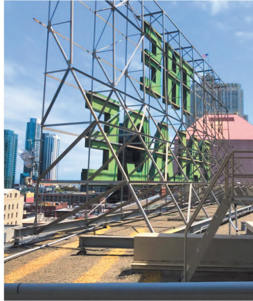
GALVANIZED STEEL FRAME WITH PARTIAL ACCESS AT FRONT AND FULL ACCESS AT BACK
